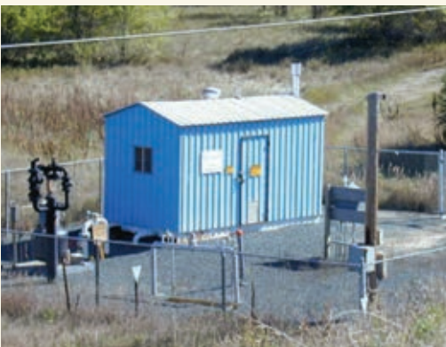
City gate meter station.
