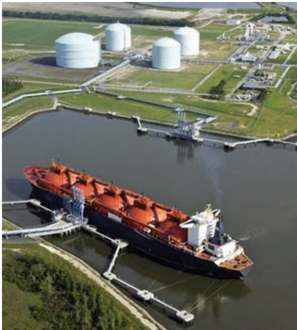
Insulated Low Pressure Storage Tanks for LNG
