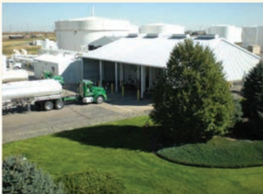
Truck loading facility.
