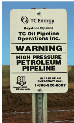
Typical TC Energy Keystone marker sign on the pipeline right of way (ROW) at road/ railway and canal crossings
