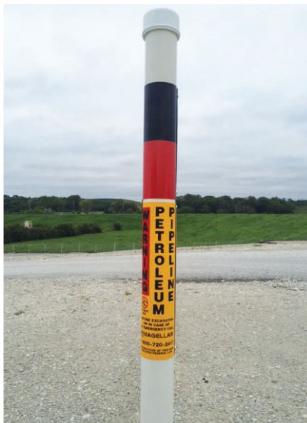
Our pipeline markers can be typically identified by the black and red bands at the top.
