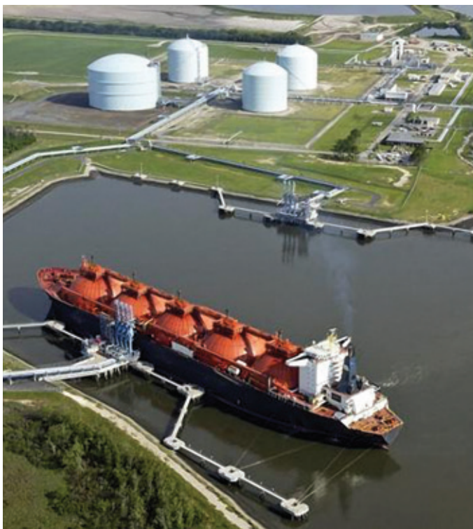
Insulated low pressure storage tanks for LNG
